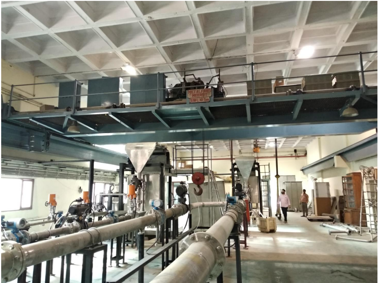
Figure 1. Photograph of the old 10 Ton Crane along with Primary Water Flow Calibration Facility
