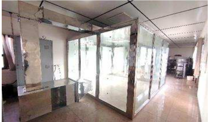
Clean air delivery rate (CADR) testing facility for air purifier
