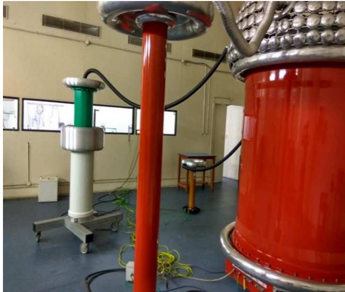
Calibration set-up for 200kV divider
